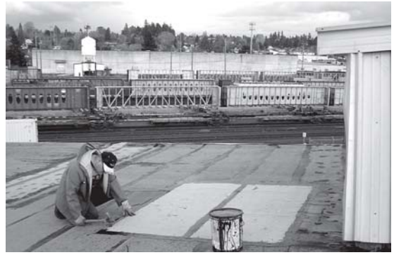
Dave Brown fixing leaks on the roundhouse roof
